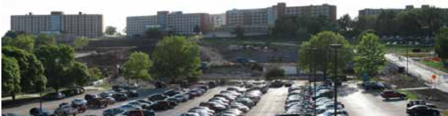
Central District construction (currently underway)
