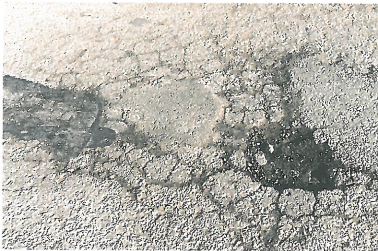
Figure 1: Pothole
